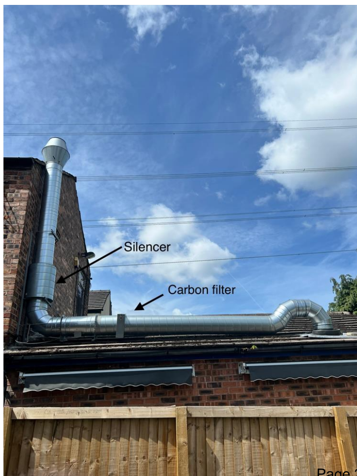
Photo 8: Extended Flue – Annotated
